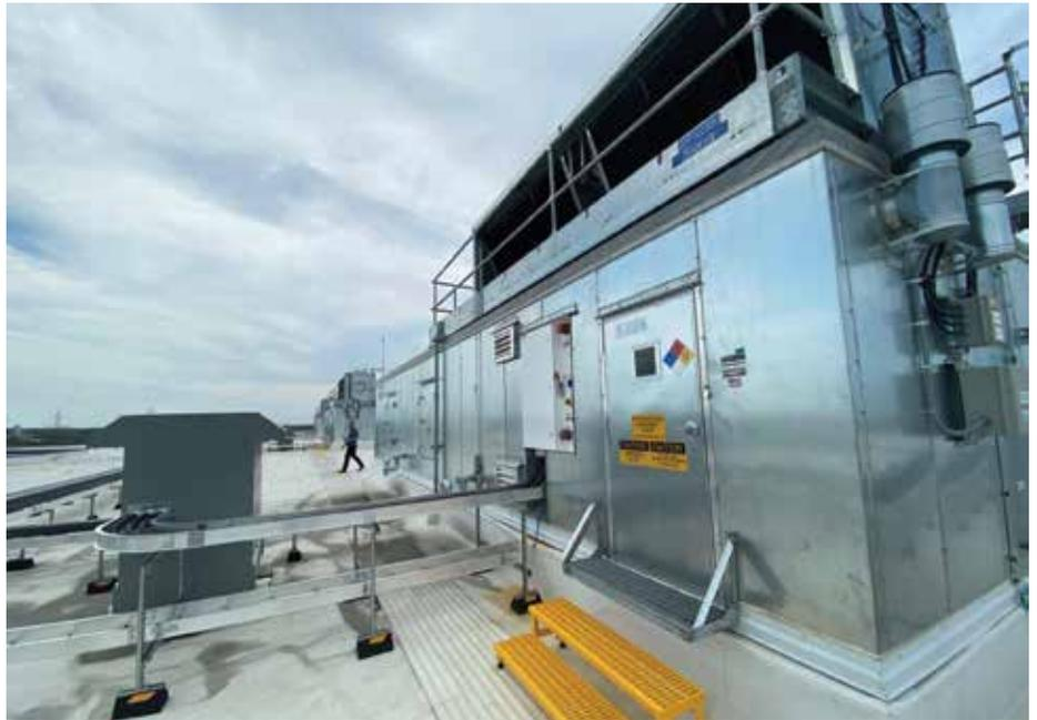
For instance, it installed Variable Frequency Drives on most of the compressors and evaporator fans to take advantage of cube-root savings.
